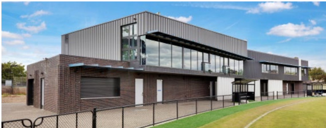
Elsternwick Park Oval 1 Pavilion
